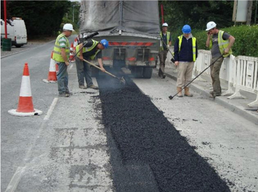
Figure 6.9: Reinstatement of Road Surface Over Trench
