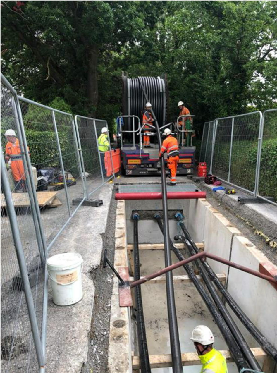
Figure 6.11: Typical Set-Up of HV Cable Pulling Procedure
