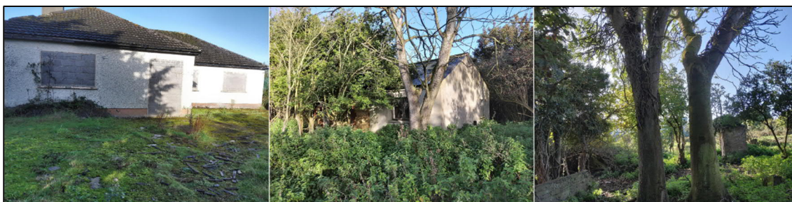
Figure 10.5: Potential Bat Roosting Sites Near the South-Western Border of the Dublin Airport, Along the Ballystruan – Forrest Little Route.
