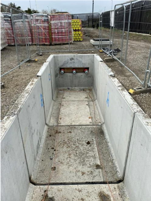
Figure 6.10: Completed Joint Bay prior to Cable Installation (pre-cast)
